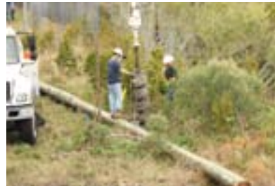
Above: Preparation for the pole installation begins with the auger, highly specialized equipment and knowledge are required to install poles. Prior to pole installation all underground utilities must be located. Photo Credit: Ed Tess
